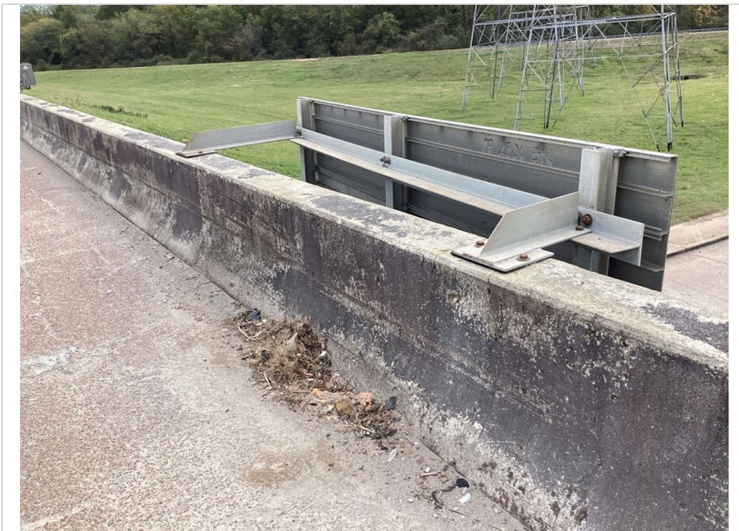
Bridge mounted sign upper connection
