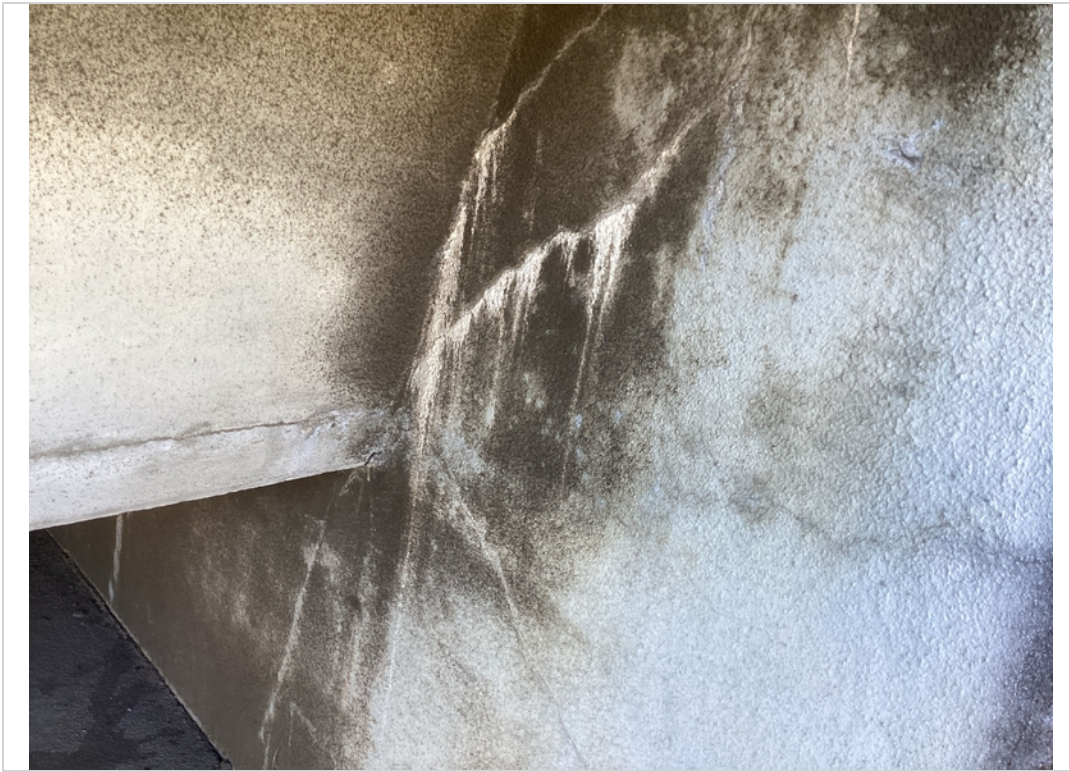
Abutment 1 crack
