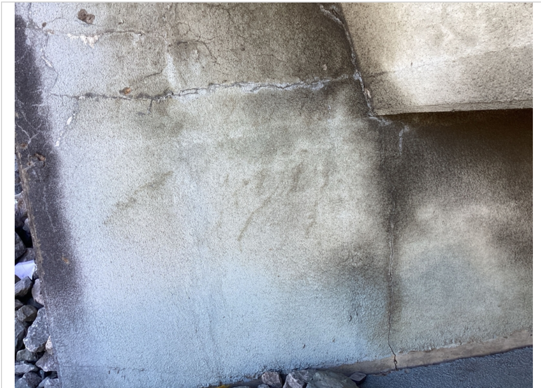
Abutment 2 , 1/8" cracks
