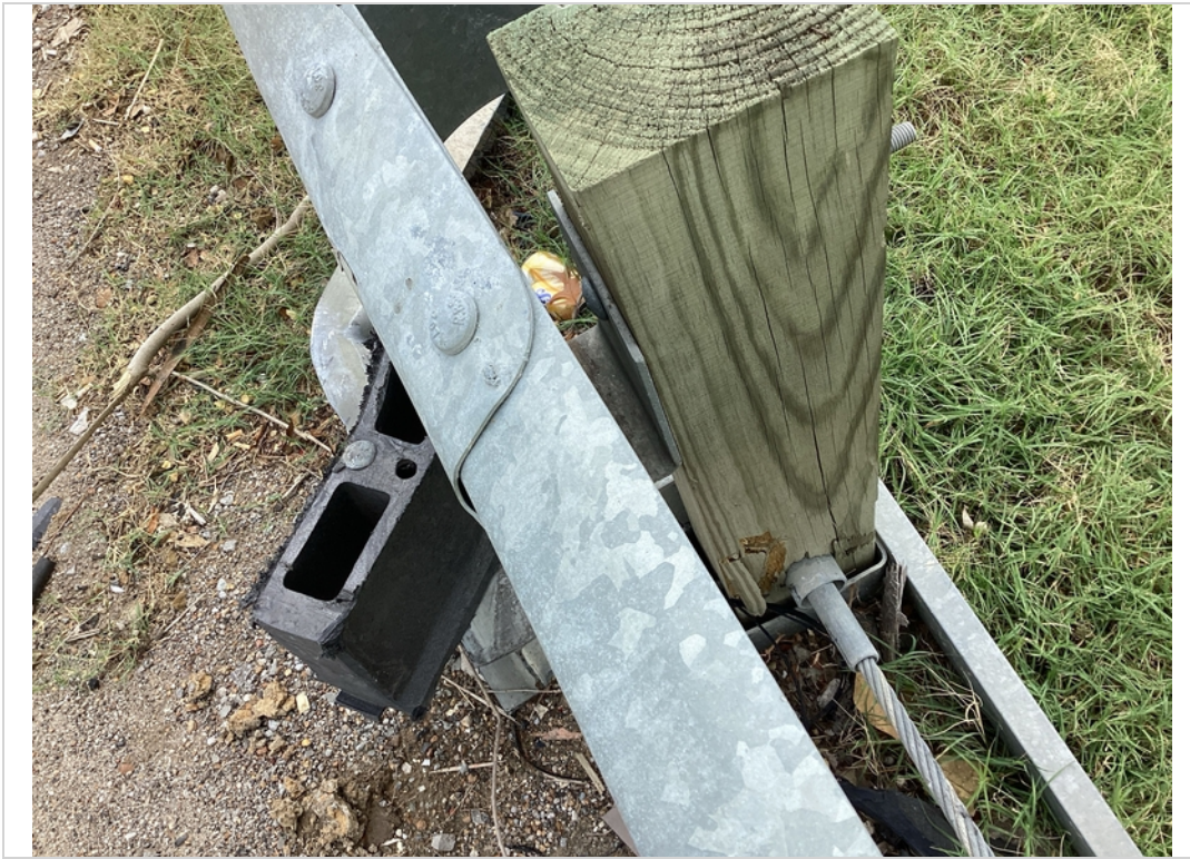
Approach 2 right terminal not attached
